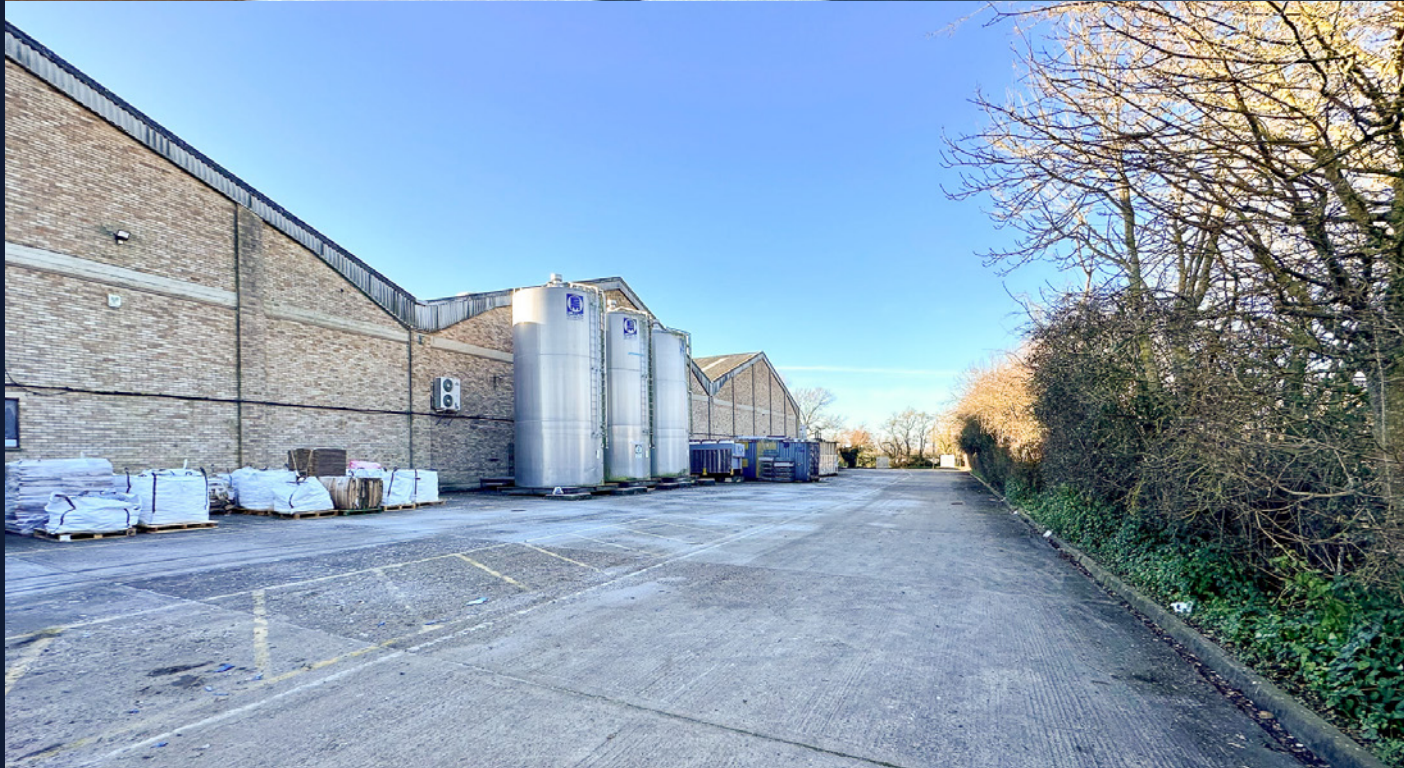
Photo of Unit A Irton House offices
